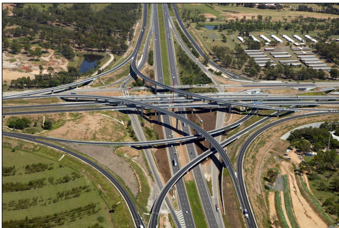
Figure 2: The Light Horse Interchange in Western Sydney (Source: NSW Roads and Maritime Services, 2013)
