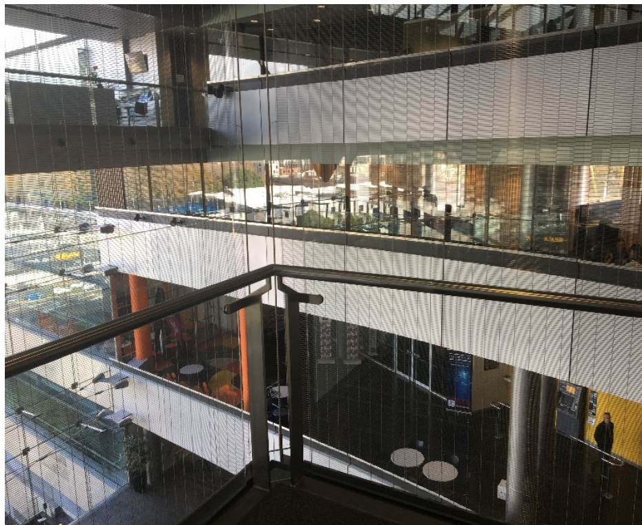
Figure 2. Wire mesh ‘death’ barriers, Owen G. Glenn Building, University of Auckland
